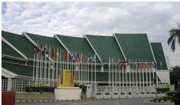
The UN building in Bangkok, which is the Asia-Pacific region's headquarter under the administrative direction of the United Nations.
